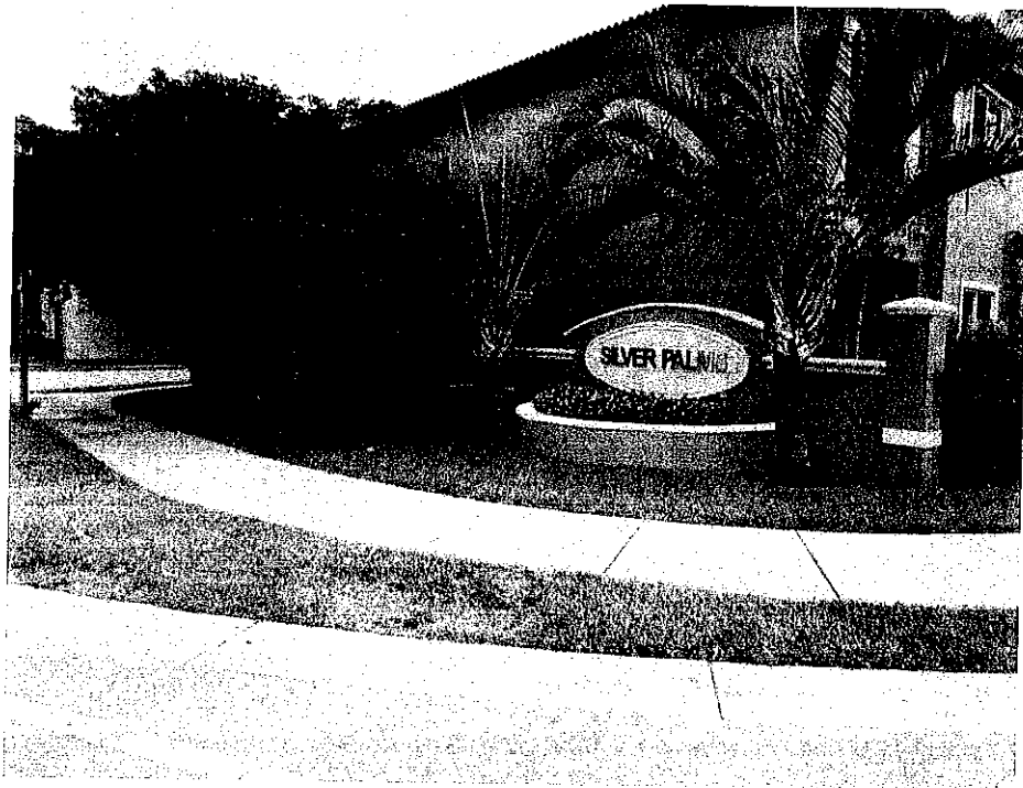
Entrance Feature Tract "A" (north of SW 230 th Terrace) – Well-maintained
