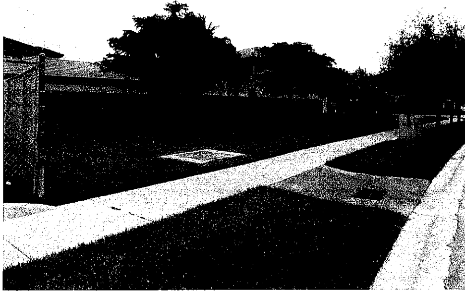
Park Tract "R" (facing northeast) – Well-maintained
